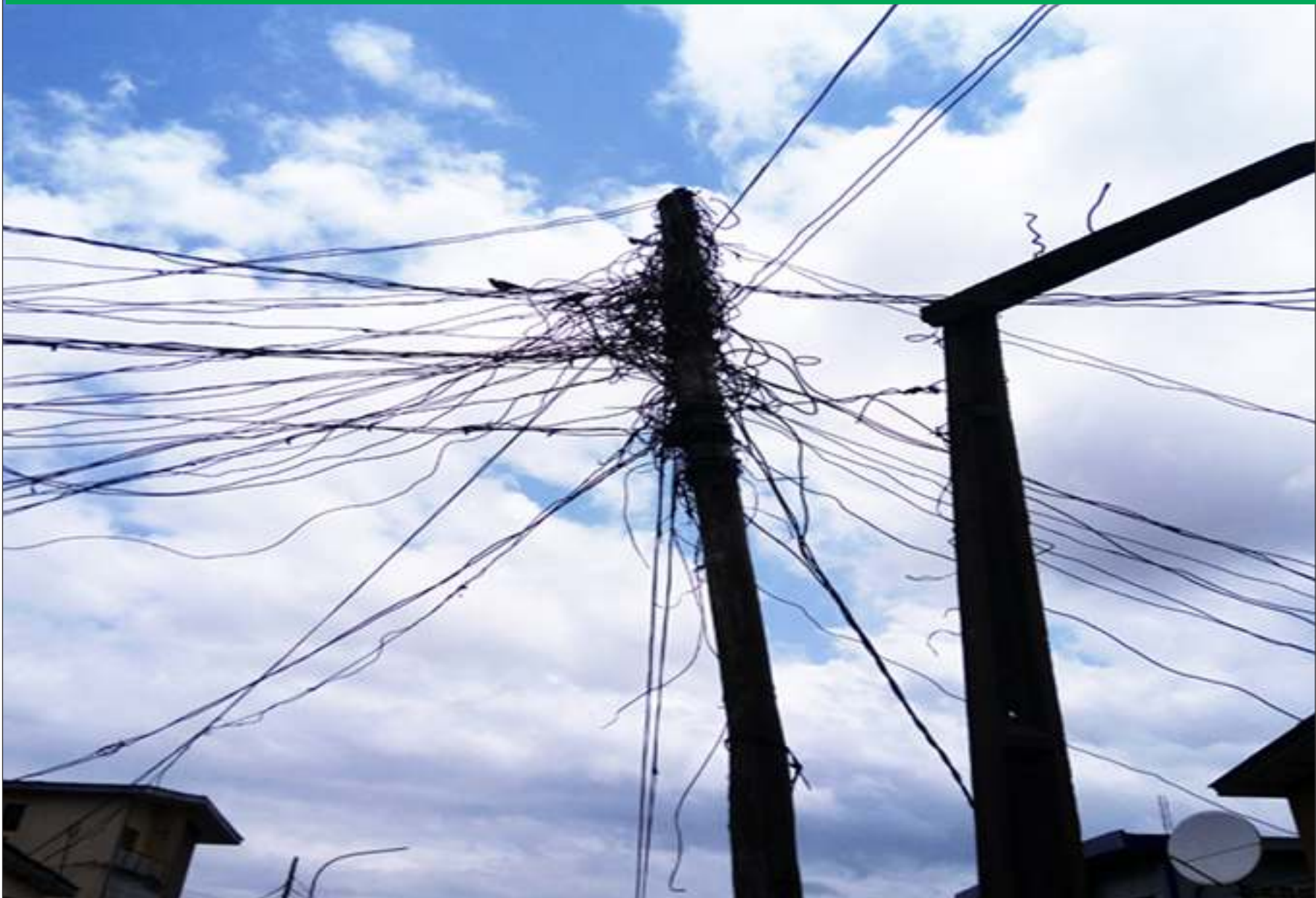
Damaged pole and clumsy cable at Unity Street, Off Toyin Street, Ikeja, Lagos
