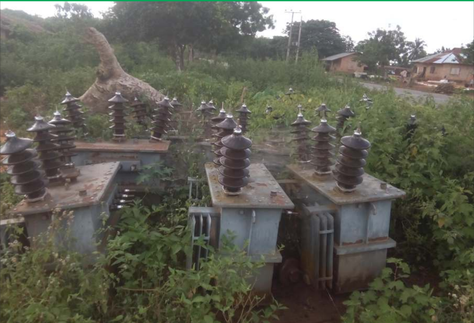
Twenty Six distribution transformers rotting away in Ologiri, near Oja-Odan in Ogun State
