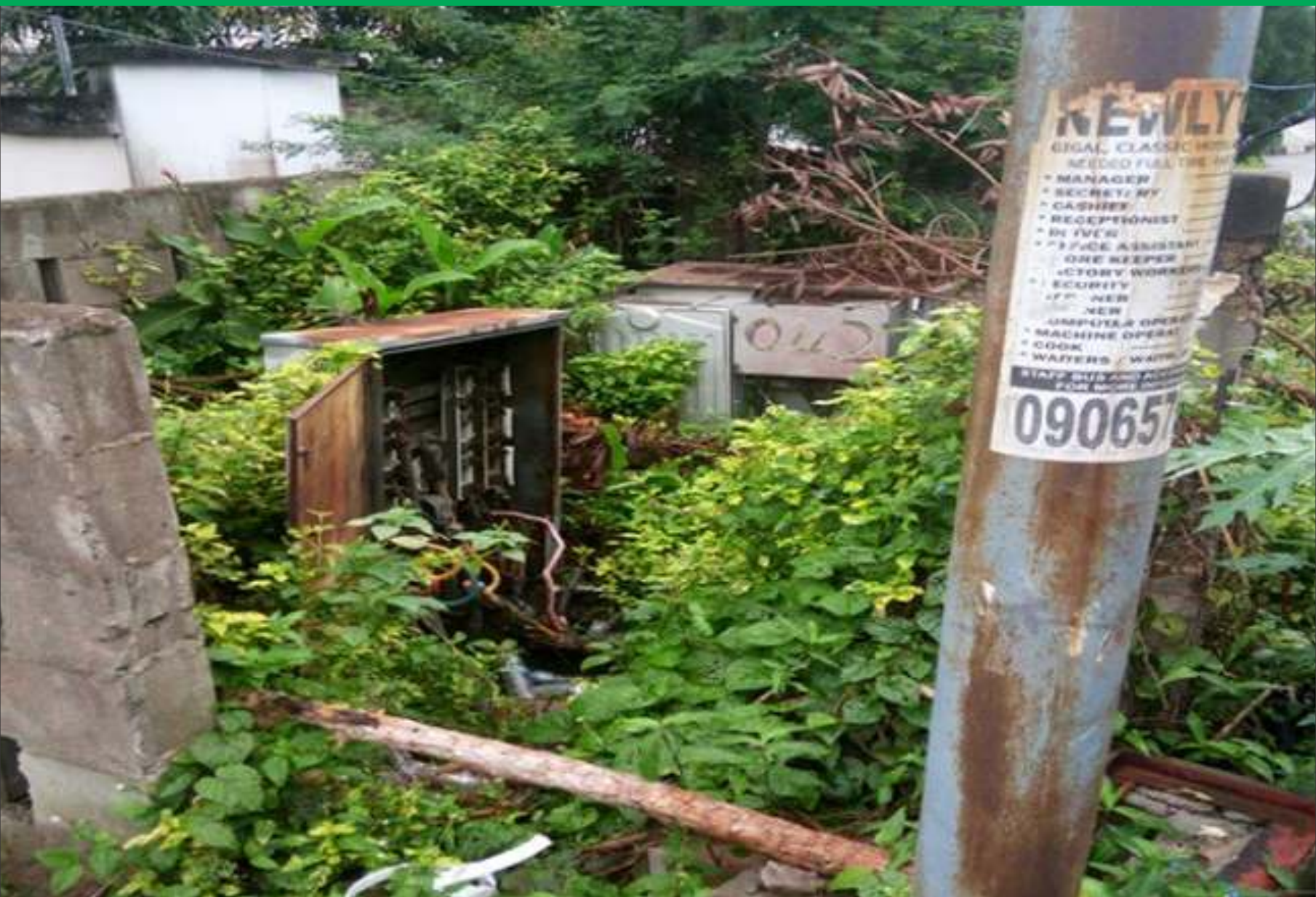
Transformer and feeder pillar at Babatunde Jose junction, Samuel Manuwa Street in Victoria Island overgrown with weeds
